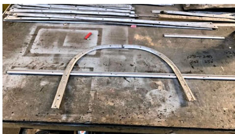
The goalpost shape aluminium trim around the Emergency door on 243 which had to be rectified so the plastic would fit. [Keith Walker]
