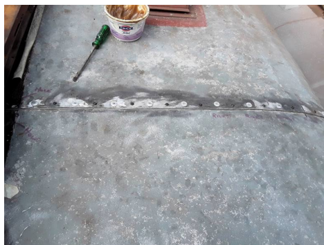
Roof panels on 262.
